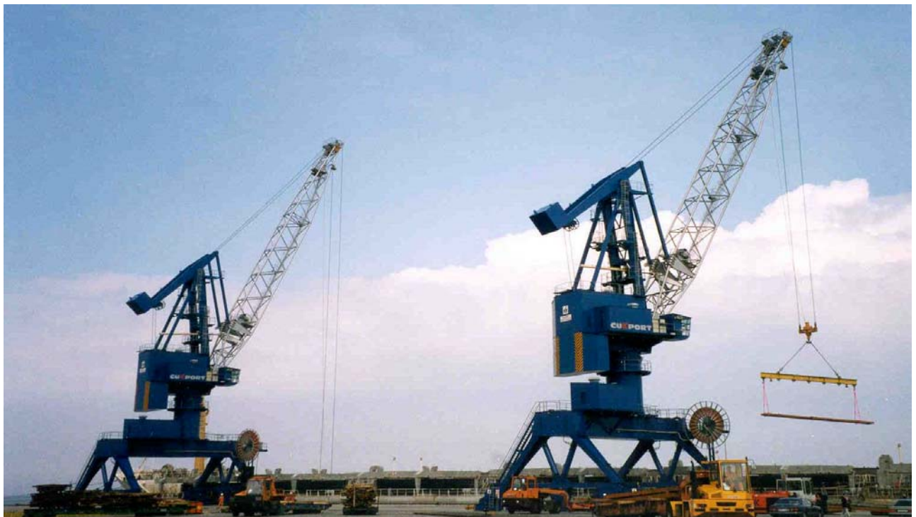
Fig. 15: New luffing cranes in Cuxhaven / Germany
