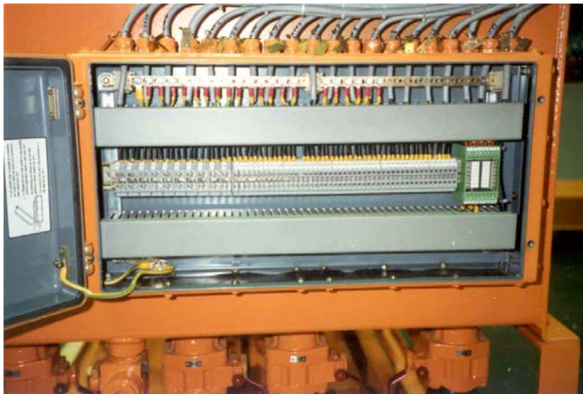
Fig. 31: Terminal box interface on the hydraulic power pack
